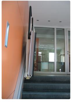
The Auto Fold feature automatically folds the platform if left unattended for a period of time at a landing (optional).
